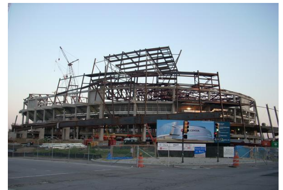
BOK ARENA under construction in Tulsa, Oklahoma
