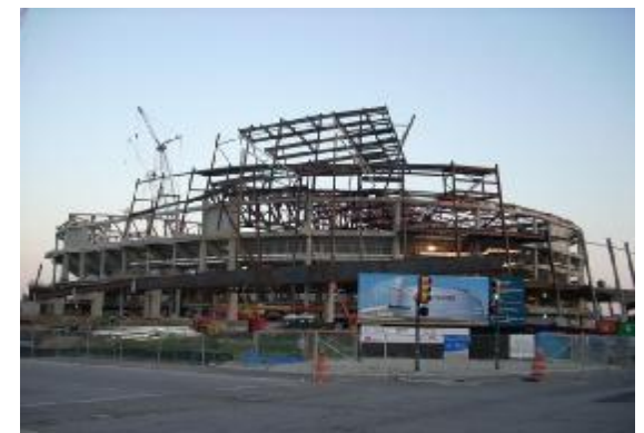
BOK ARENA under construction in Tulsa, Oklahoma
