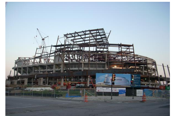
BOK ARENA under construction in Tulsa, Oklahoma
